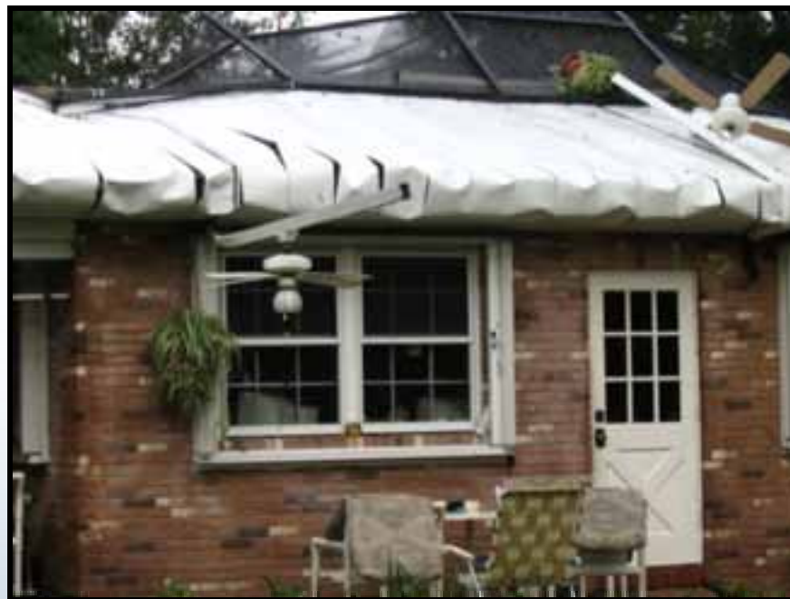
Tornado damage in Brandon
